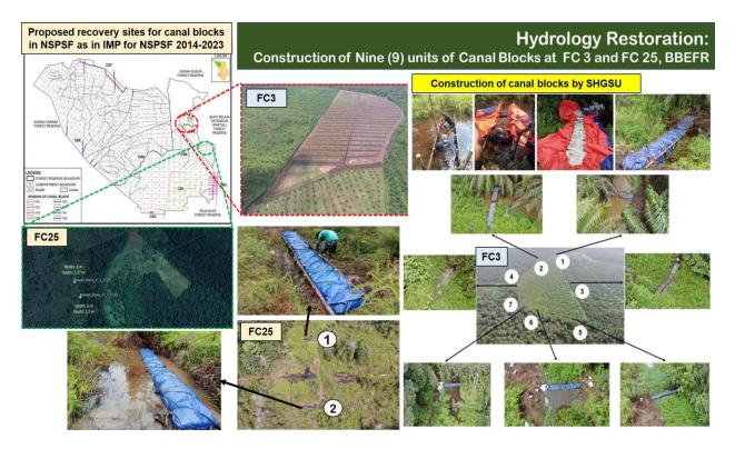
Figure 8. Construction of nine units of canal blocks at FC 3 (7 units) and FC 25 (2 units), BBEFR
